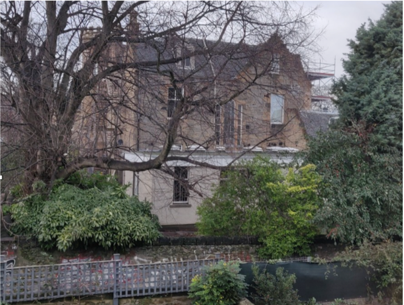
Figure 3. View of 10 Chalmers Cres extension from 15 Mansionhouse Rd, showing its the proximity to the gardens across Lovers Loan and the poor screening of the trees. The roof terrace would be above where the skylights are now, on top of the beige box.
